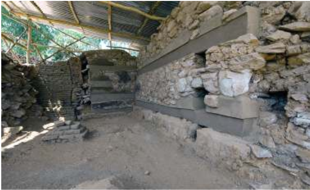
Fig. 15a: One room of the Grat Be'al Gebri after the restoration of the timber-frame construction (DAI, Irmgard Wagner)
