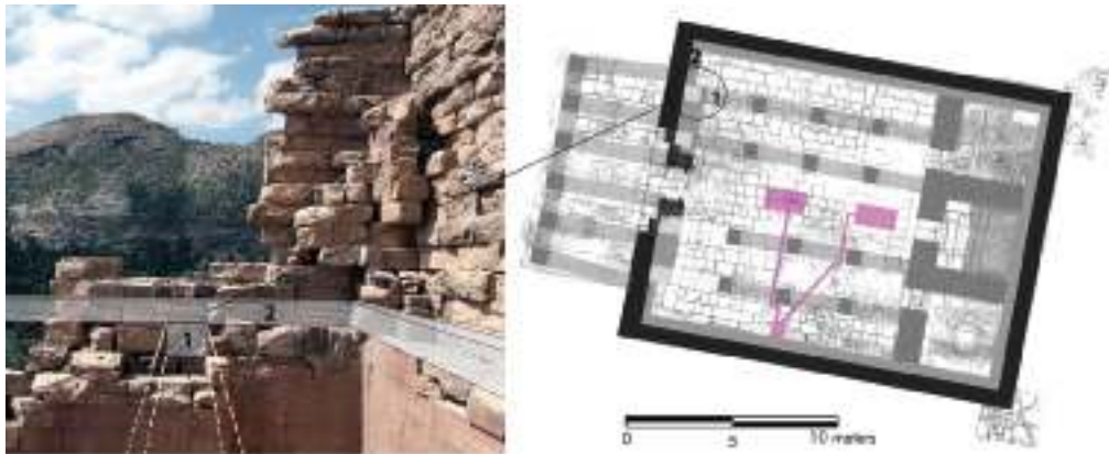
Fig. 13. Large beam holes (1) in the walls M4 and M5, lying below the circular wall projection, mark the position of the first order of the ceiling beams.
