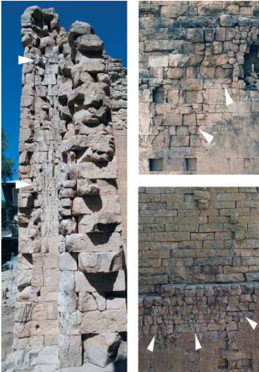
Fig. 3. The inner façades of the Great Temple and its damage caused by conflagration.
